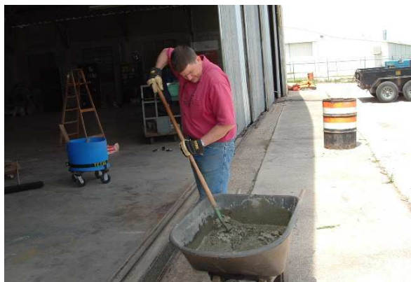
"Hangar Mother", David Bradshaw mixes cement for the H3 door threshold.
